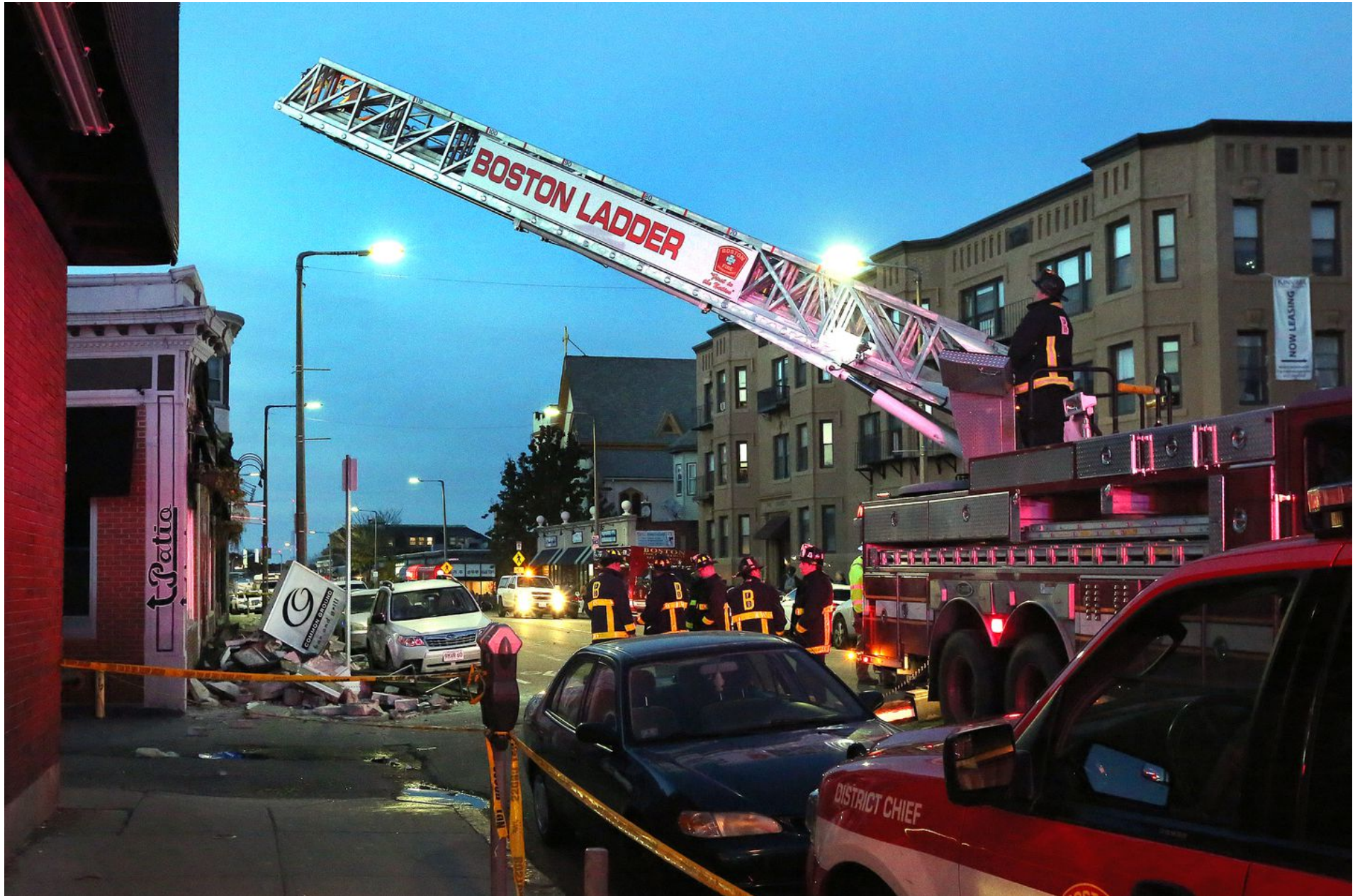
The aftermath of the facade collapse on Nov. 4, 2018 PAT GREENHOUSE/GLOBE STAFF
