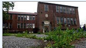
Community center begins to take shape
