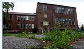
Community center begins to take shape
