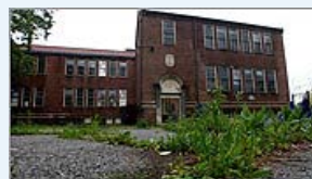
Community center begins to take shape
