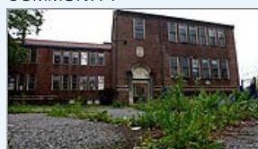
Community center begins to take shape
