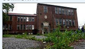
Community center begins to take shape
