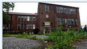
Community center begins to take shape
