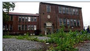
Community center begins to take shape
