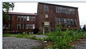
Community center begins to take shape
