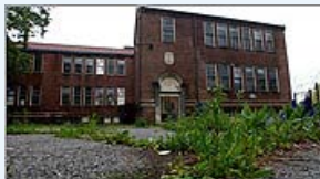
Community center begins to take shape
