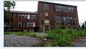
Community center begins to take shape
