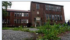
Community center begins to take shape
