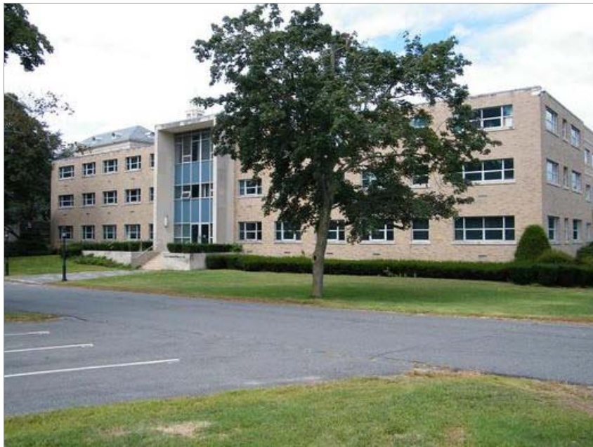
The former Archdiocese of Boston Chancery building at 2121 Commonwealth Ave. in Brighton is expected to undergo a year-long renovation beginning in January.
